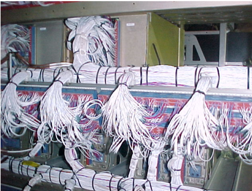
Figure 1. Typical wiring from the back of the electronics rack of an in-service transport aircraft.
